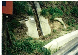
Slope protection subsidence
