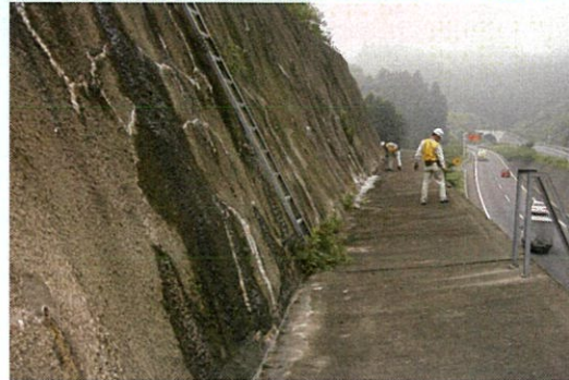
Visual inspection of slope gradient
