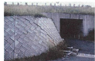
Slope collapse of embankment slope
