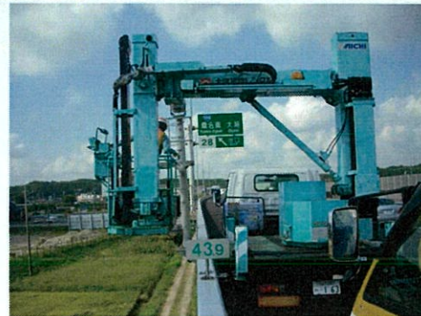
Structural examination of lighting facility
