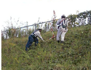
Visual inspection of slope gradient
