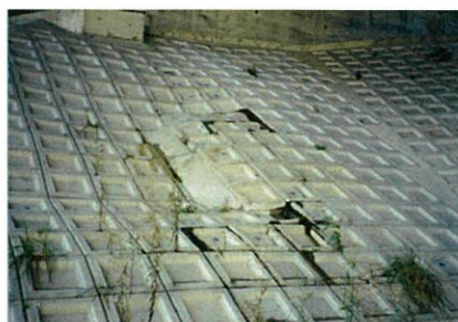
Slope protection subsidence
