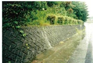
Slope protection subsidence
