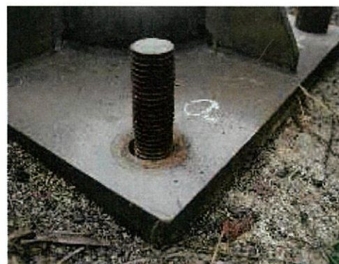
Corrosion and thinning of anchor bolt
