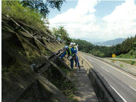
Visual inspection of excavation slope
