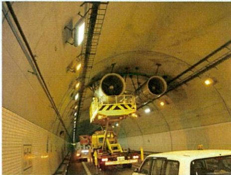
Structural examination of tunnel ventilation facility
